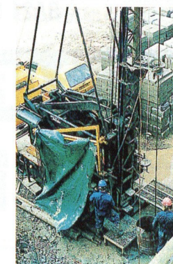
>> A drilling rig sinks a borehole for the new ground's water supply
